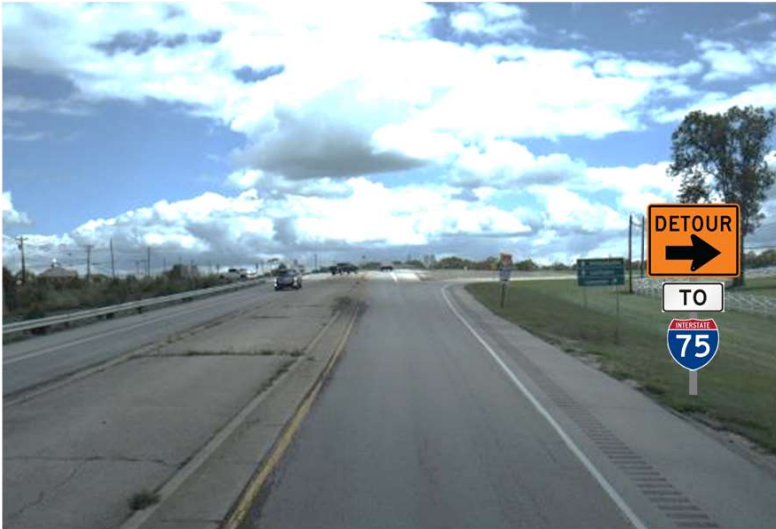
Detour Signage Eastbound KY 29
