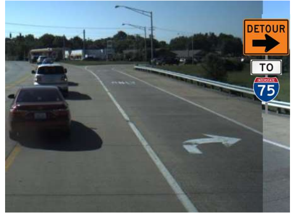
Detour Signage for Westbound Bypass Rd.
