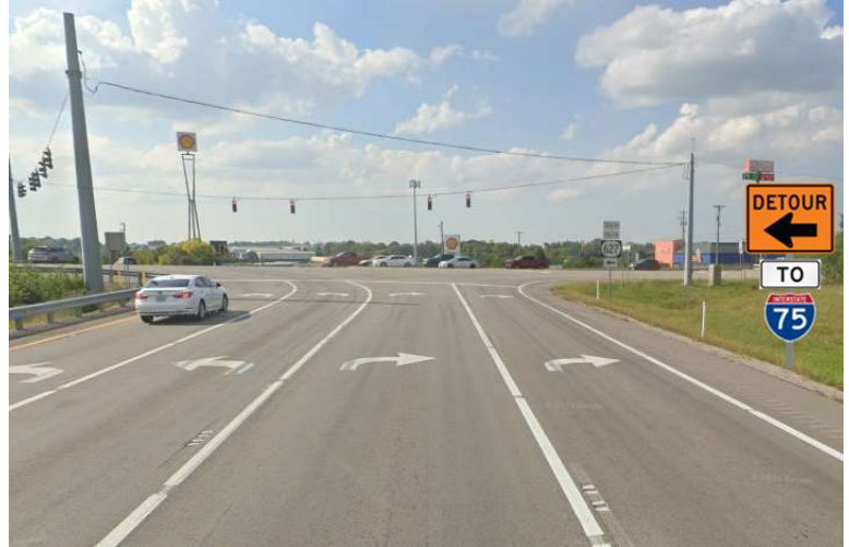
Detour Signage for Westbound Off-Ramp
