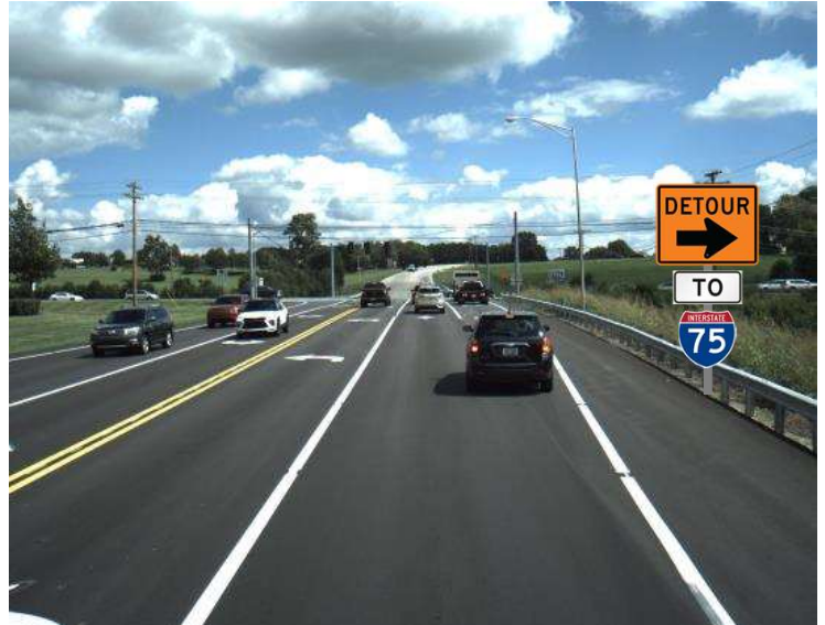
Detour Signage Eastbound KY 169
