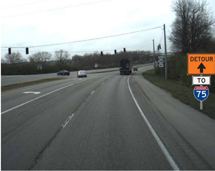
Detour Signage for Southbound US 127
