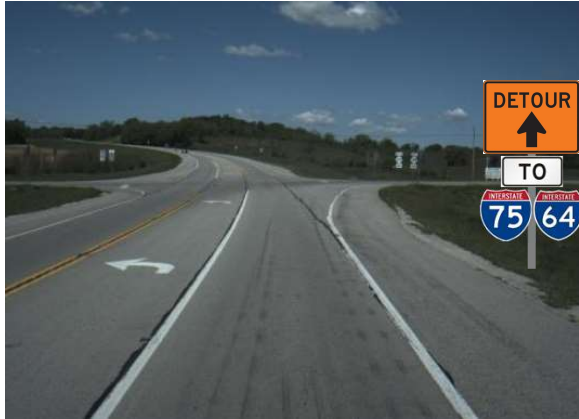
Detour Signage for Westbound US 150
