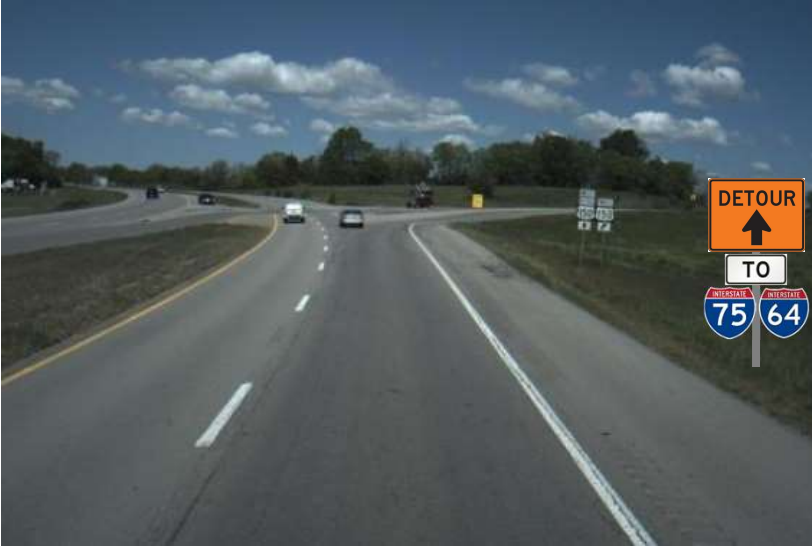
Detour Signage for Westbound US 150
